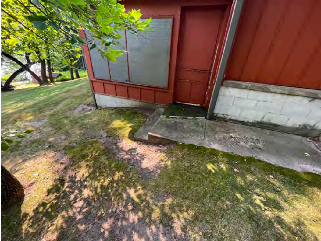
Drainage from existing structure
