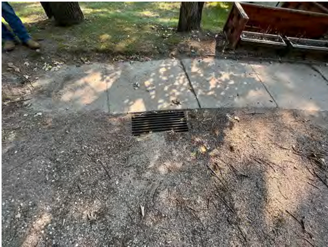
Storm drain located on the property.
