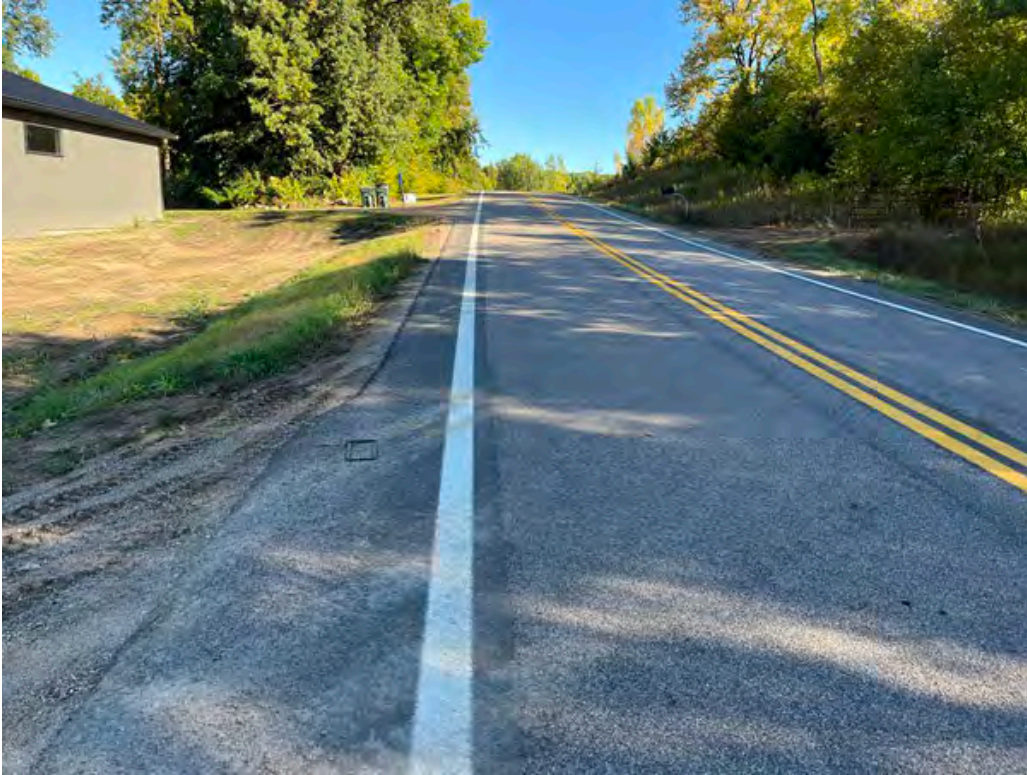
Looking north down Alcott Drive
