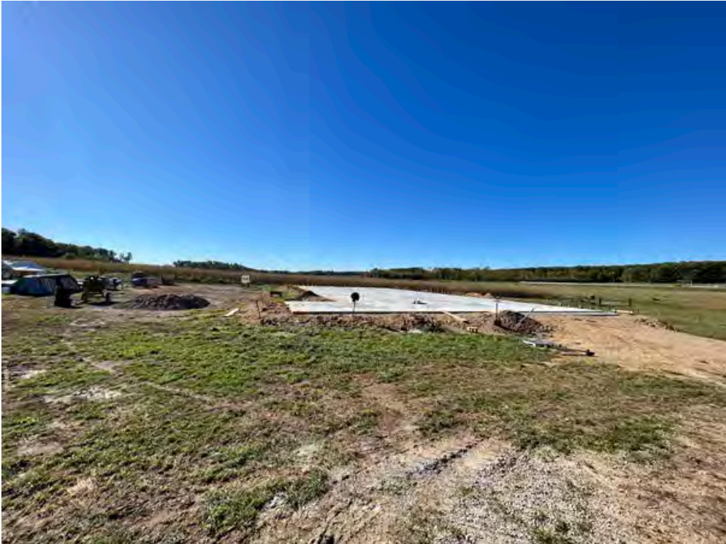
Proposed building site
