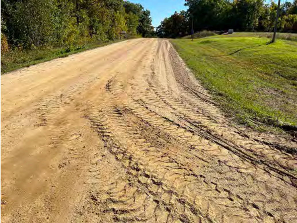
Looking east down 464 th St from east driveway
